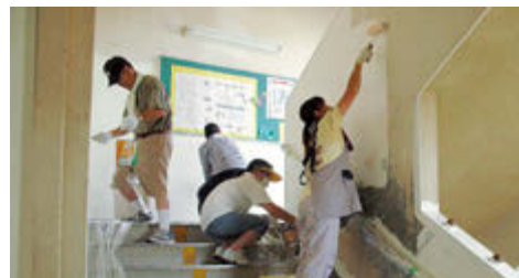
保護者と地域の皆さんによる小学校の校舎の補修 (学校応援団) The school repairing by the parents of the elementary school students and the locals (School Supporters)
